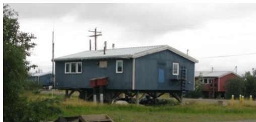
Photo: Most houses and utilities in rural Alaska are built above ground to avoid digging into permafrost
